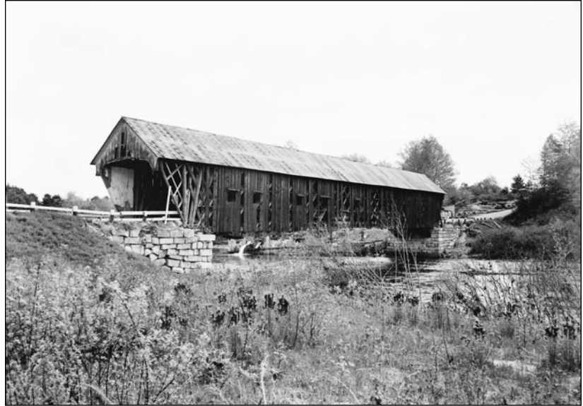
Fig. 4. Henniker Road Bridge, spanning Contoocook River, Hopkinton vicinity, New Hampshire, 1862, destroyed 1936, John Briggs, designer (Library of Congress, Prints and Photographs Division, Historic American Buildings Survey, HABS NH, 7-HOPV, 2-1).
