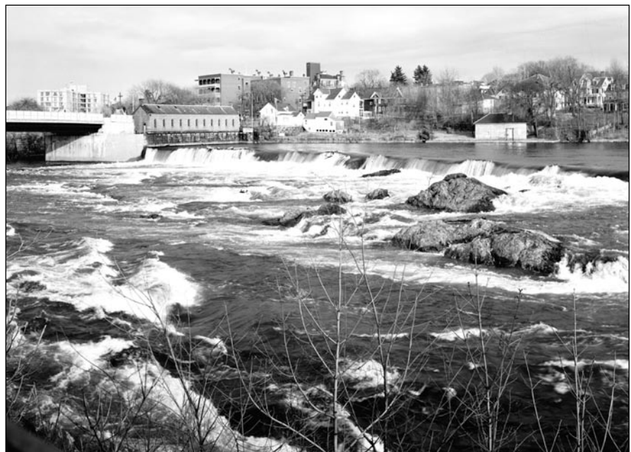
Fig. 2. Pawtucket Dam and Gatehouse, Merrimack River, Lowell, Massachusetts, 1875, designer unknown (Library of Congress, Prints and Photographs Division, Historic American Engineering Record, HAER MASS, 9-LOW, 8A-12).
