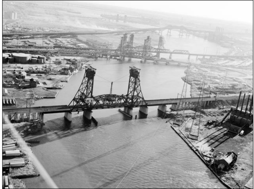
Fig. 7. Vertical lift bridges, Hackensack River, Kearny, New Jersey, early twentieth century, John Alexander Low Waddell, designer (Library of Congress, Prints and Photographs Division, Historic American Engineering Record, HAER NJ, 9-KEAR, 2-3).
